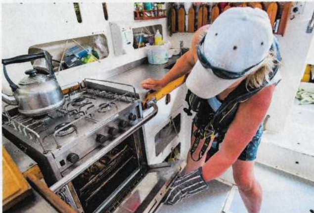
Domestic systems for cooking and heating can be equally as important as mechanical systems
