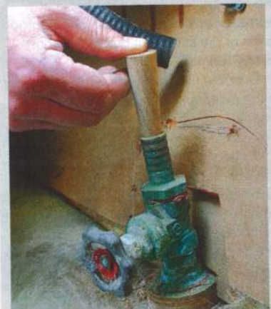
Keep a selection of tapered softwood plugs handy to seal pipes or holes
