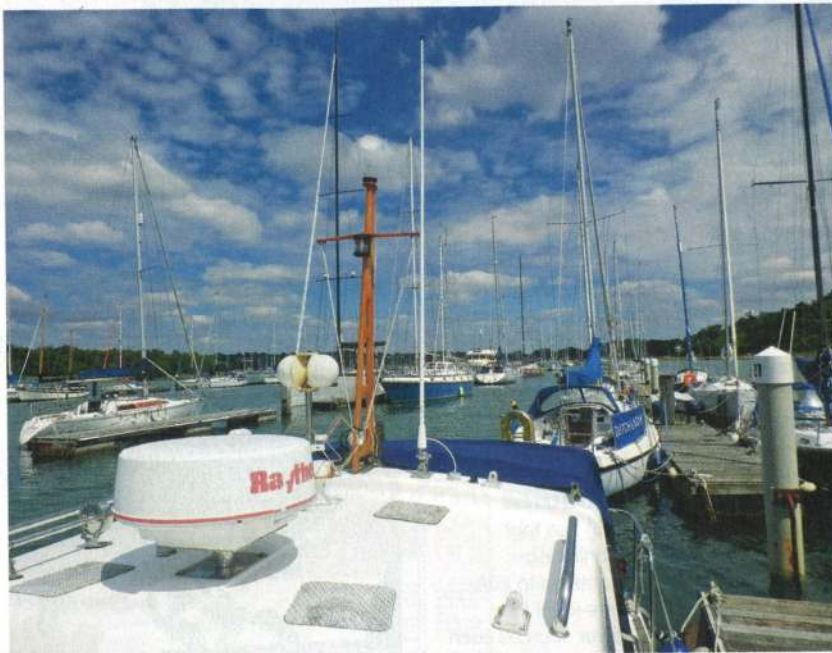
1 The removal of various old antennas left mounting brackets and cable glands which needed to come off too.
