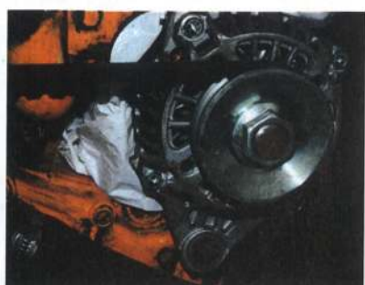
Temporary plastic deflects seawater leak away from the new alternator
