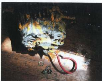
Seawater and alternators don't mix... this one has had it
