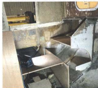
Engine box and chart table carpentry will be completed in the winter
