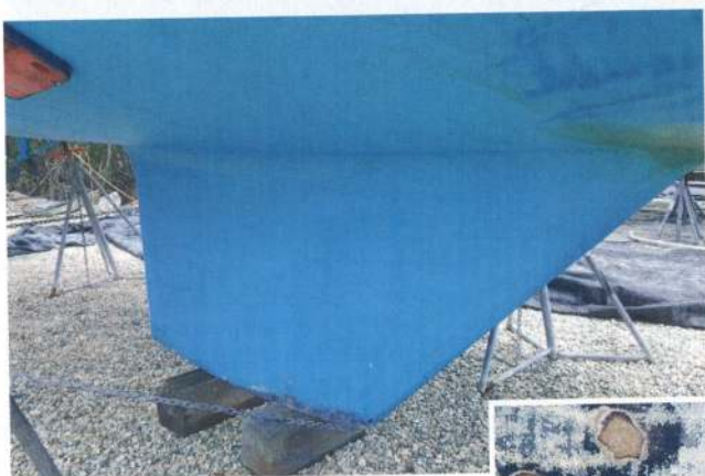
Bolt-on lead keels with stainless steel bolts should be rebagged if over 20 years old with signs of separation or weeping
